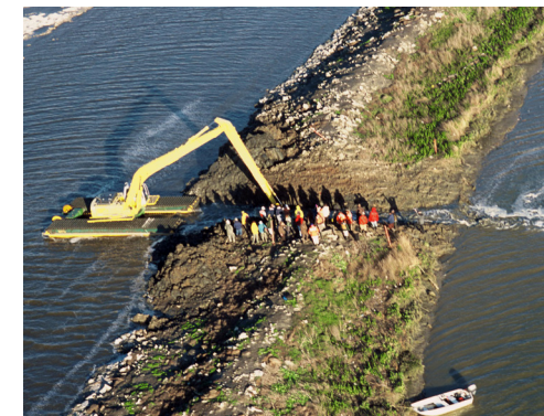
South Island pond breach in South SF Bay.
